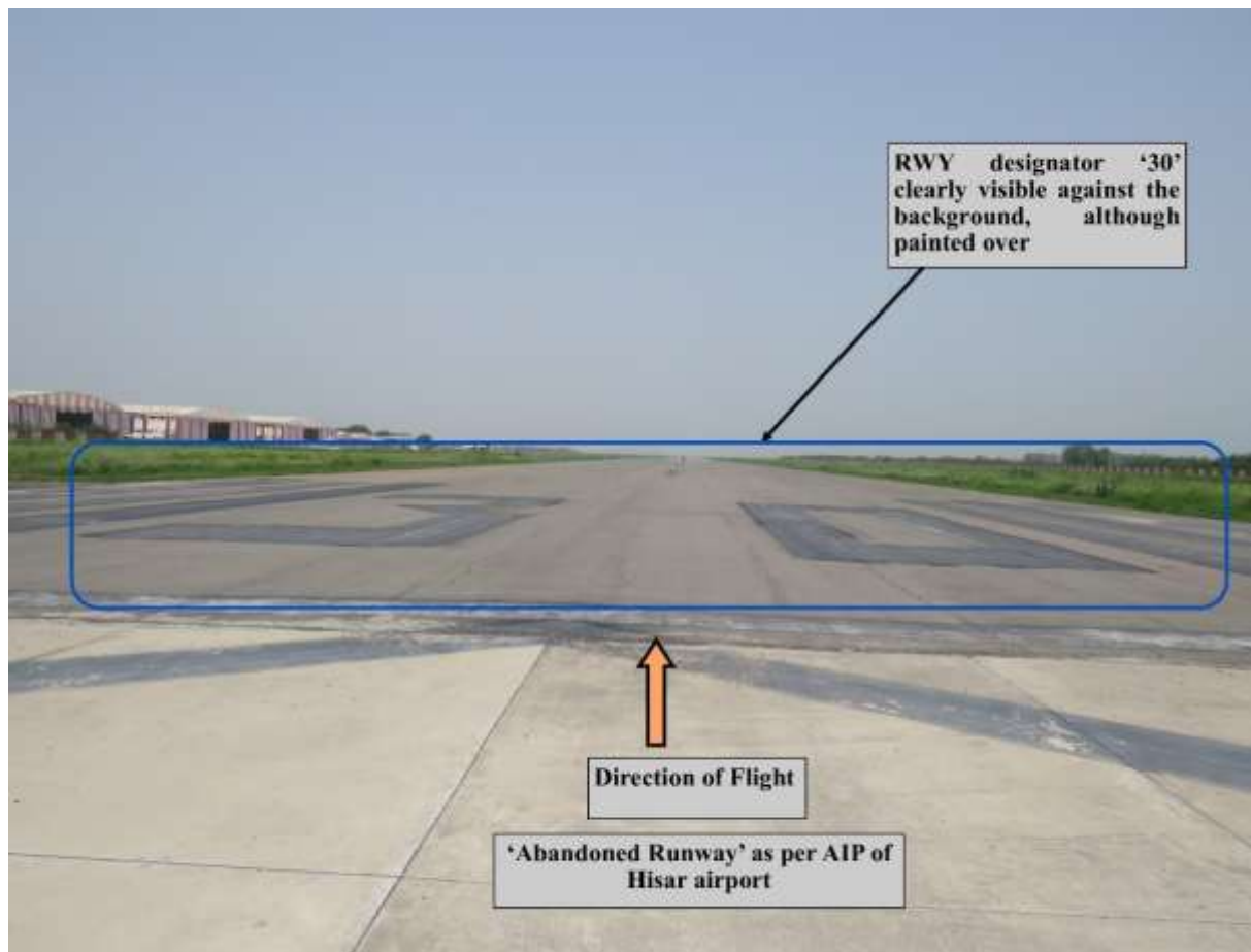
FIG 8: 'Abandoned Runway' portion ahead of RWY30
